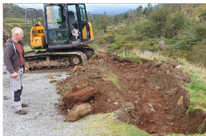
Fig. 6: Graving for fundament
